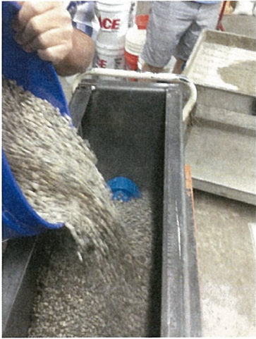
pea gravel being poured into box
