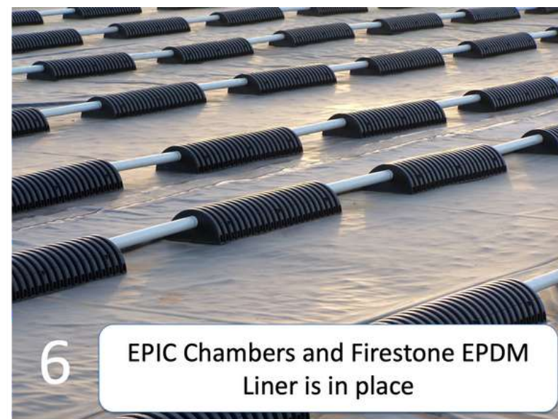
2 Laying the Epic Geomembrane Liner (EPDM or LDPE) Epic Recommends using Firestone EPDM Liner
