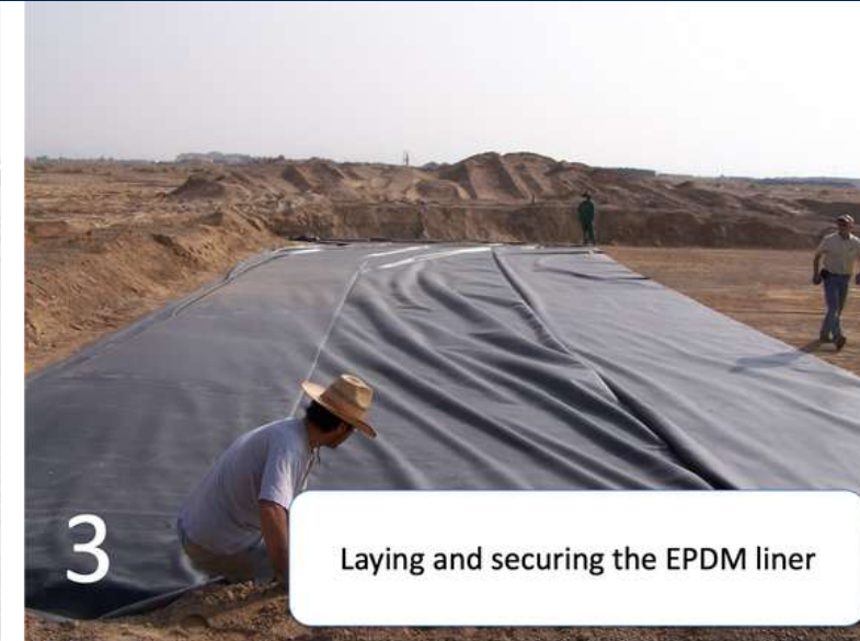
2 Laying the Epic Geomembrane Liner (EPDM or LDPE) Epic Recommends using Firestone EPDM Liner
