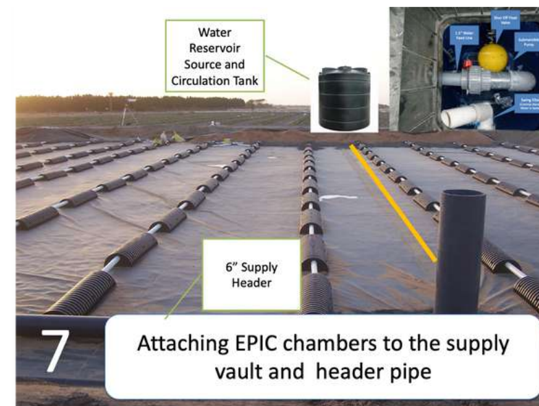
6 EPIC Chambers and Firestone EPDM Liner is in place
