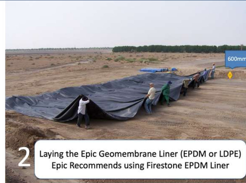
3 Laying and securing the EPDM liner
