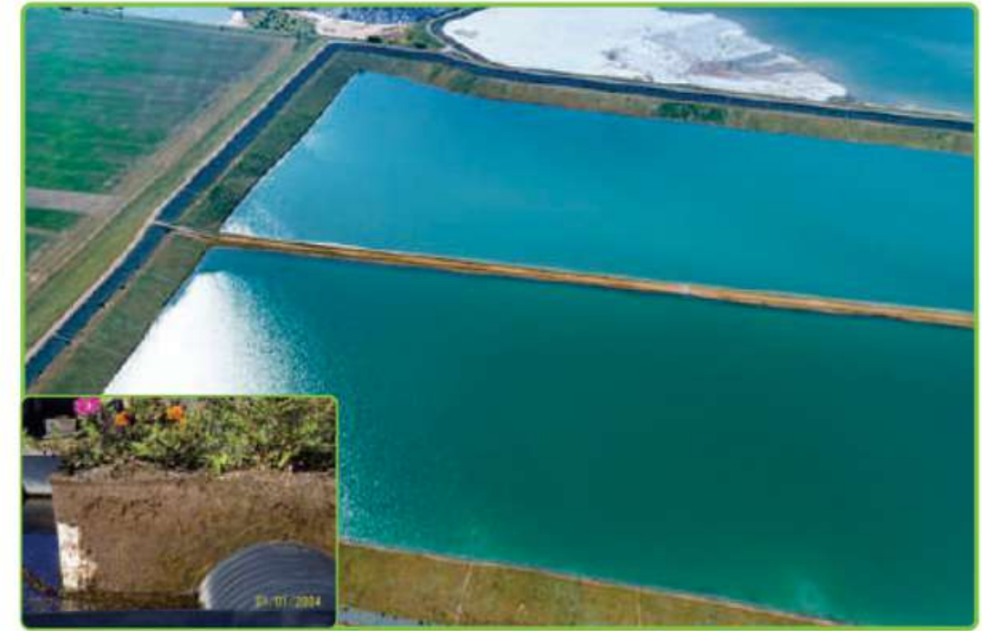
BIOFILTERING PRODUCED WATER FOR AND IRRIGATING SURROUNDING LANDSCAPE
