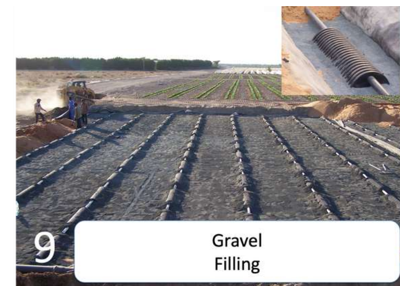
5 Installing the EPIC Chambers
