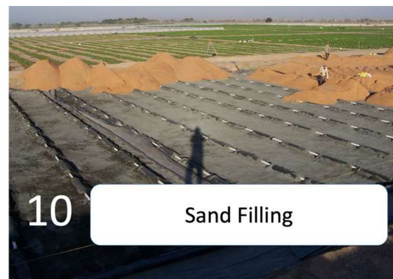
6 EPIC Chambers and Firestone EPDM Liner is in place
