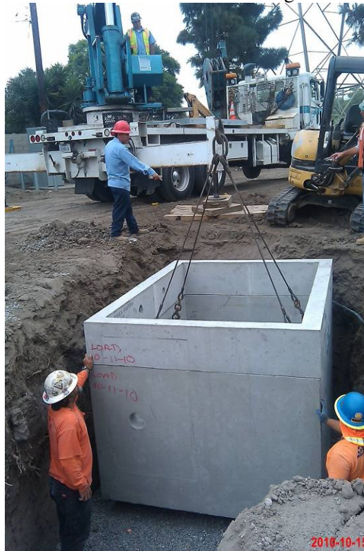
Photo was taken on October 2010. Picture of the treatment train installation.
