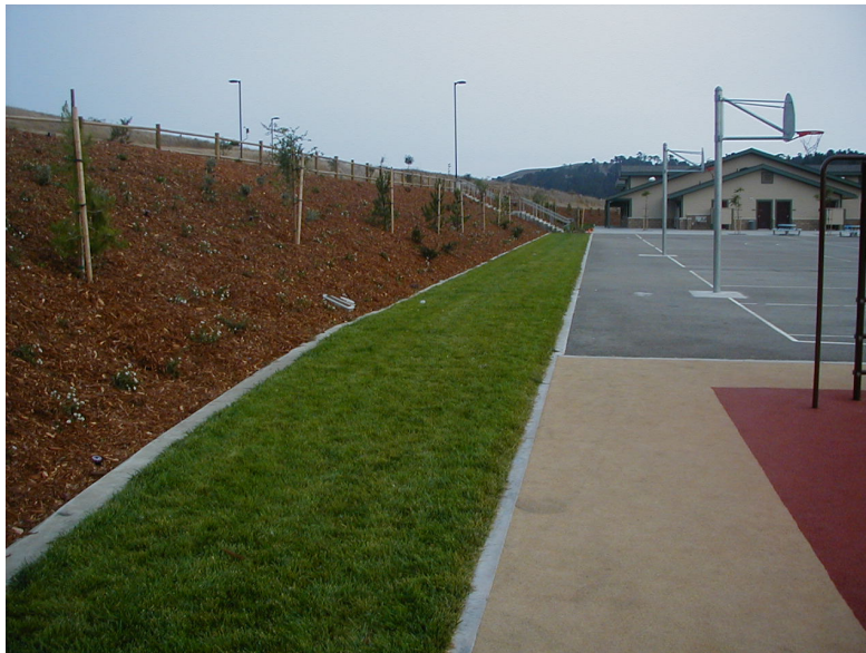
Cambria School runoff filtration and water harvesting strip at mid section.(Sipaila)
