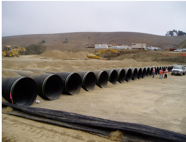
Cambria Elementary School, Storm water collection and Storage system under primary play field. (RRM design)
