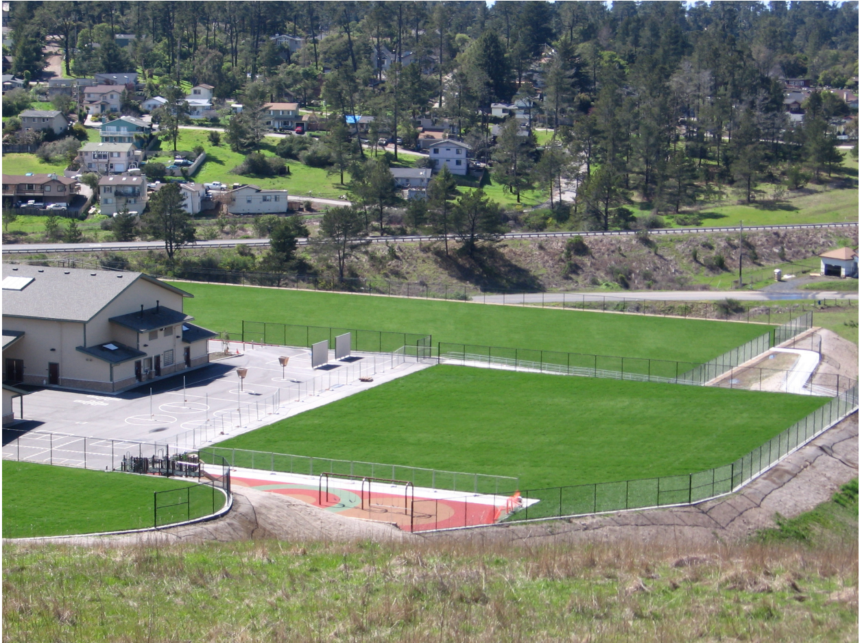
Completed Cambria Elementary Fields. Note flat laser level design of fields on tiered campus levels. (Sipaila)
