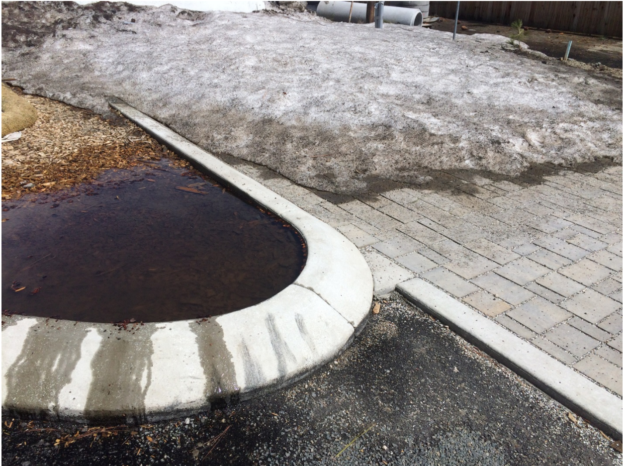
Fig 8. No soil absorption and overflow left side – vs. quick absorption in Paver area right side
