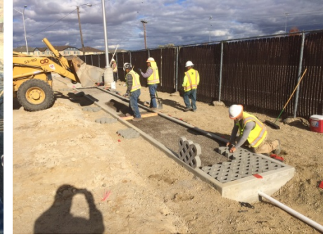
Gravel fill vibra-tamped and capped
