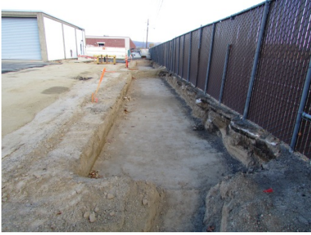
Cavity excavation in native soil
